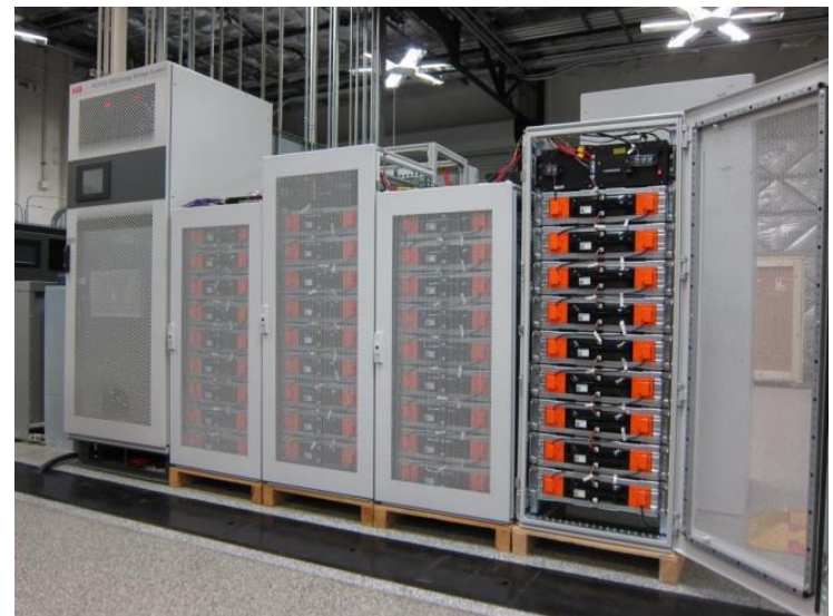
SCE Tehachapi plant, 8MW, 32MWh.
