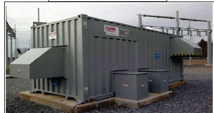
FIAMM 222-kWh System Duke Energy Rankin Substation
