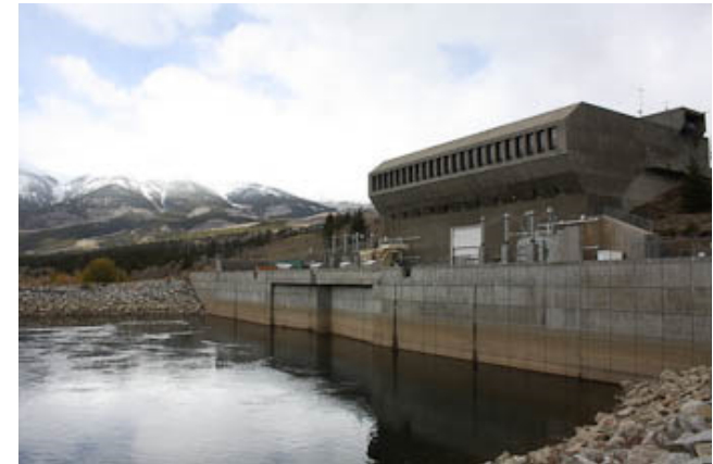
Mt. Elbert Pumped Hydro, 0.2MW, peaking plant, operational 1981.
