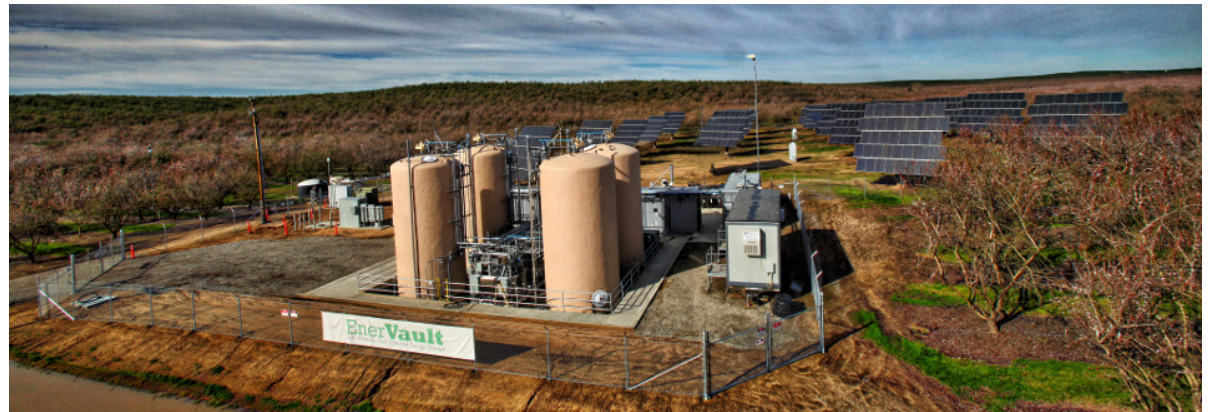
EnergVault plant, Turlock, CA. 250kW, 1 MWh.
